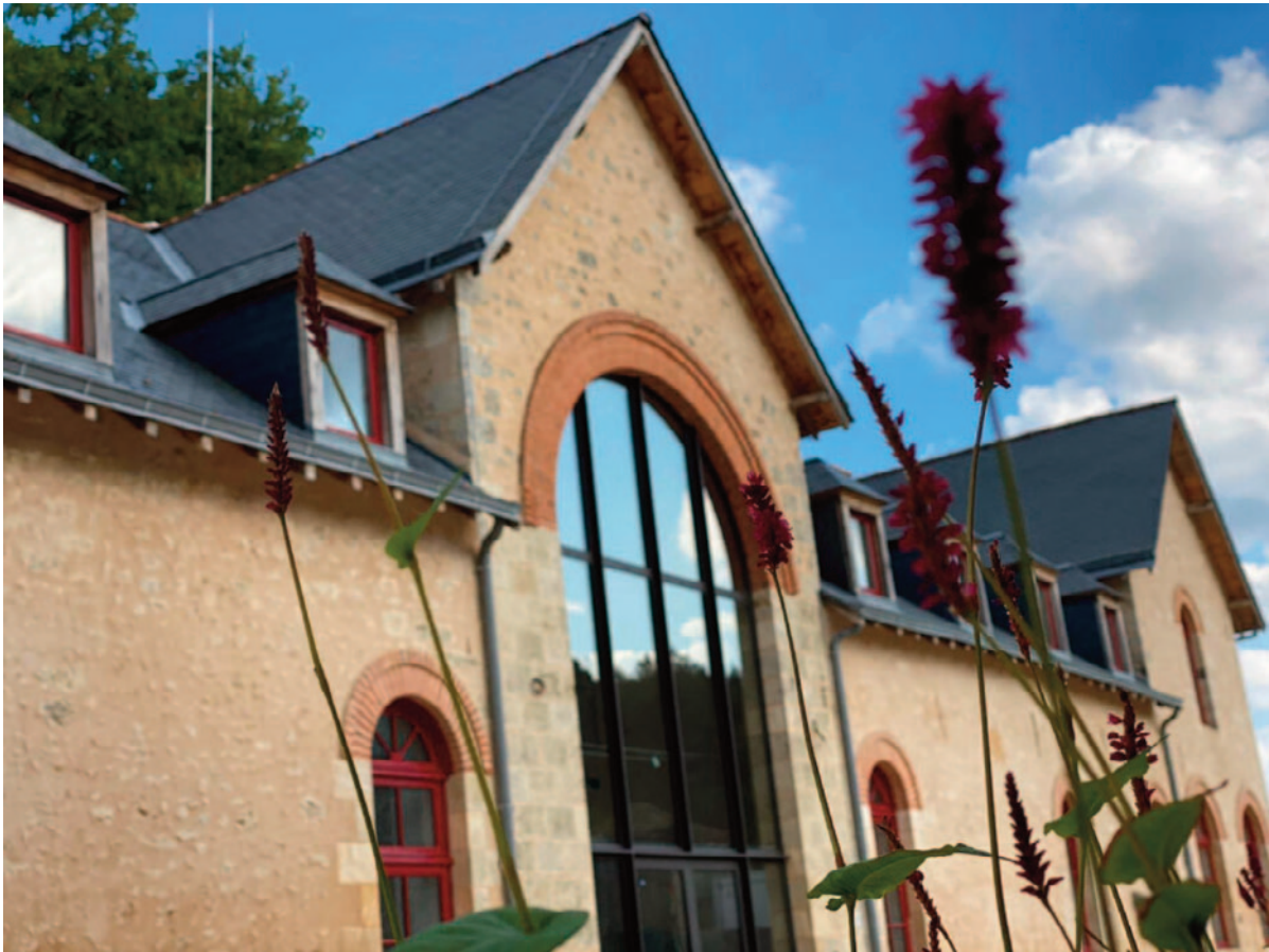
The Stables, Accomodation at Bonnevaux, France. Photo from the Bonnevaux website.
